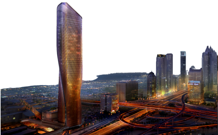
Wasl Tower, UAE
