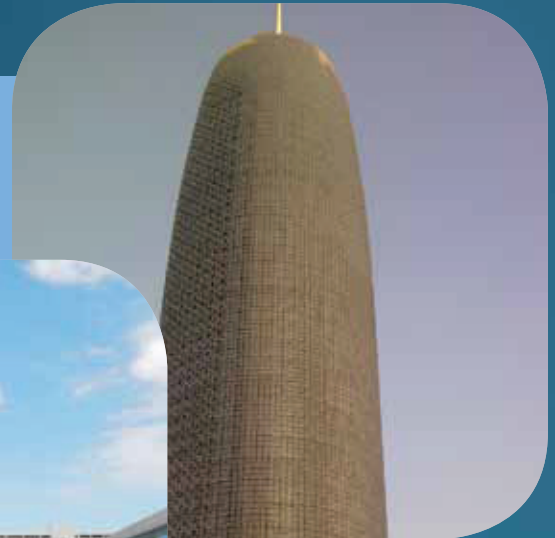
Doha High Rise Tower (Qatar)
