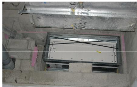
ISONE® fire dampers, as per stringent European standards **EN 1366-2**, are ensuring **2 hour fire resistance without any heat transfer and smoke leakage** (EIS 120 – 500Pa\*).
