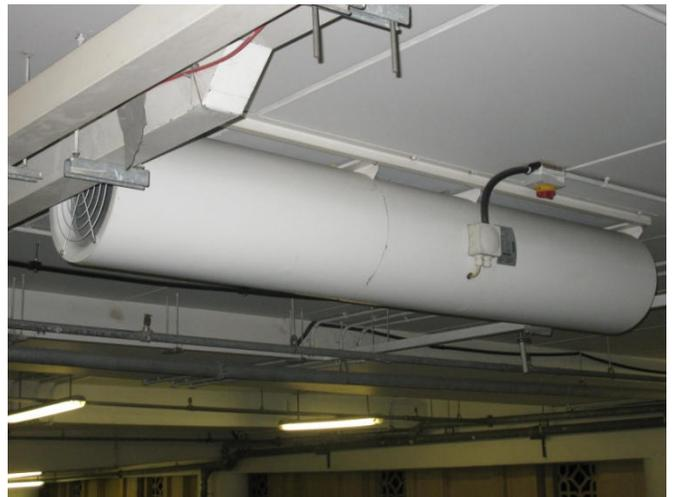
Beams and obstructions directly facing a jet fan (airflow directed on the left – cf arrow on the jet fan) – Dubai Mall (Dubai)
