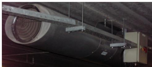
One of the main reasons behind the introduction of this system for car park application is **to avoid the constraints due to the bulky ductwork** (supply & extract ductwork removal) to guarantee:
