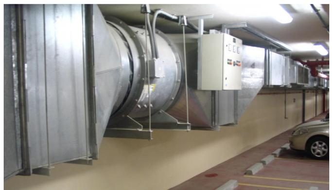
Enclosed car park – Smoke exhaust axial fan & smoke exhaust duct
